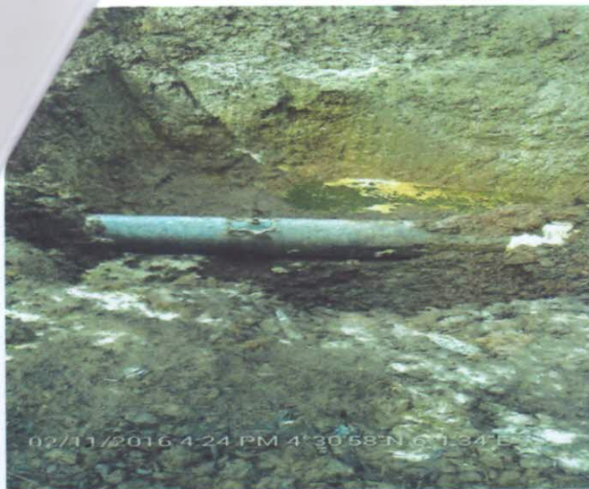
Figure 1: Cut-off Nipple on the pipeline.
