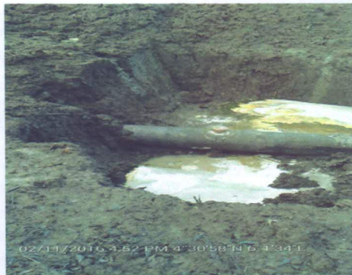
Figure 2: Coned after repair on the Pipeline .
